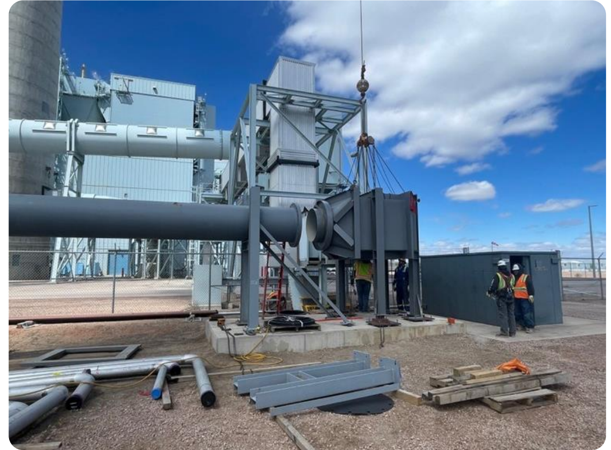
ITC tie-in and transition section
