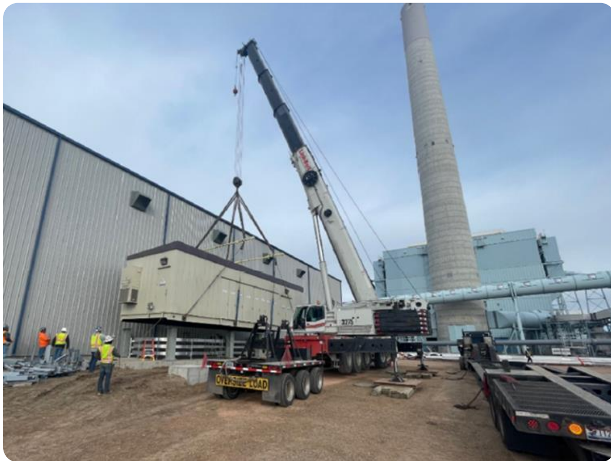
Placement of PDC building
