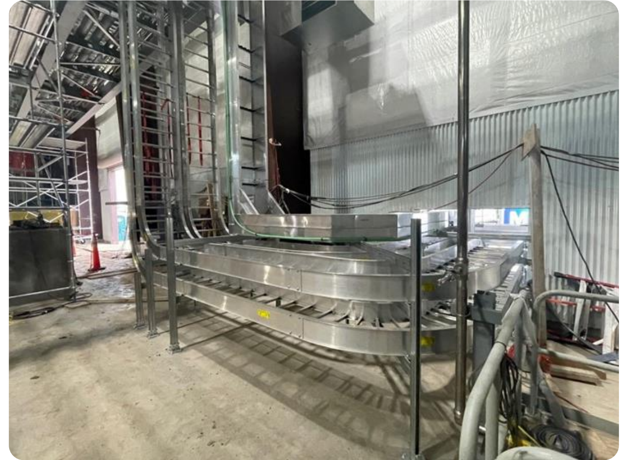
Cable tray waterfalls and penetration towards PDC building
