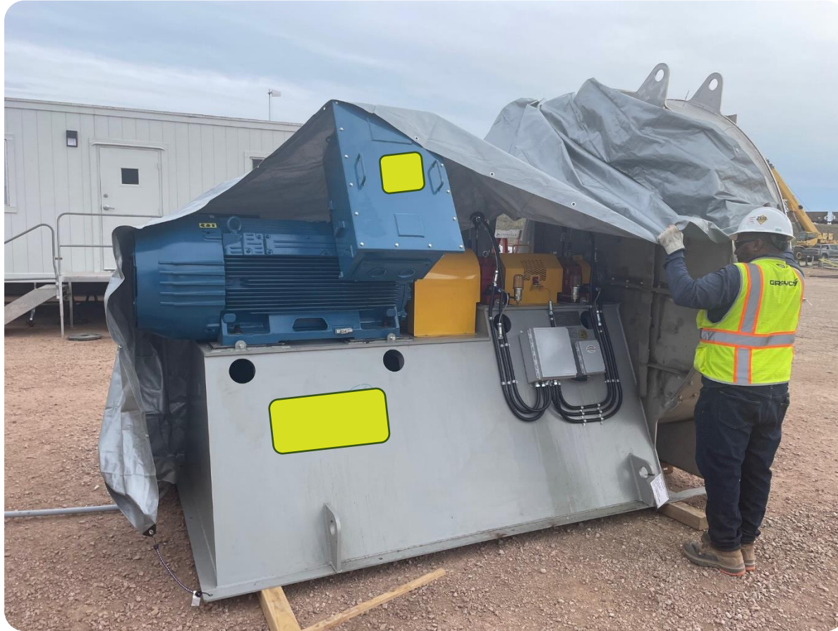
Process Equipment arrives – Flue gas blower
